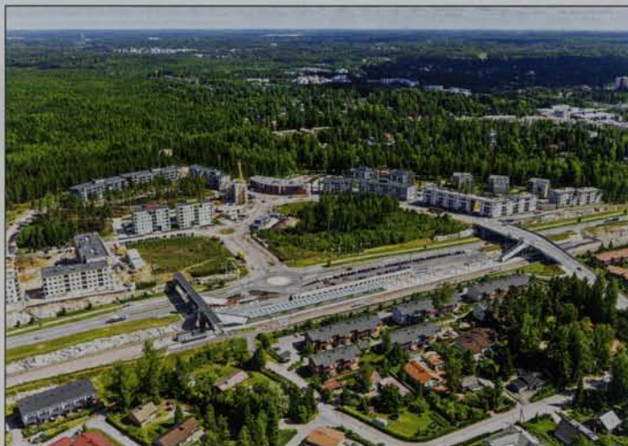
To the east of Helsinki airport the Kehärata comes to the surface before Leinelä station. Note the hard rocky nature of the sub-strata, which meant that the construction of the new railway involved a lot of blasting.
